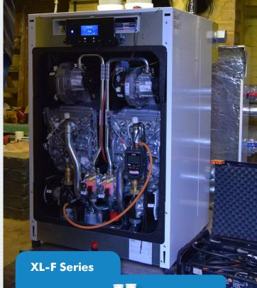
The XL-F offers outputs of 70 to 200kW from a single boiler and up to 1.6MW in cascade. All models benefit from an excellent footprint to power ratio for greater flexibility.
